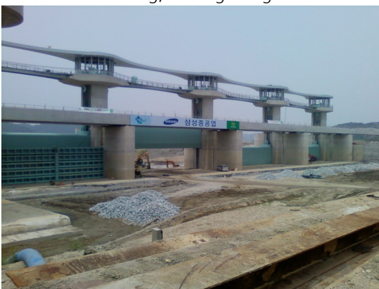
Fig 1: Floodgates under construction
