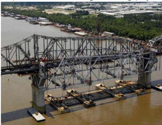
Fig 1: Huey P. Long Bridge, Mississippi River
