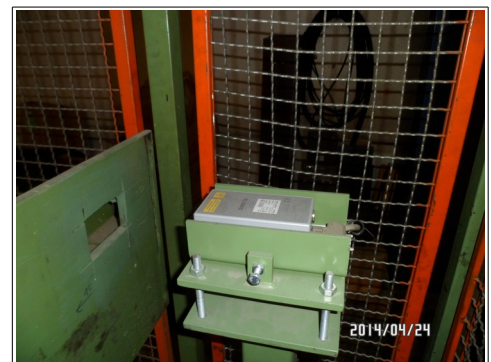
Pic 2: Installation of Sensor
