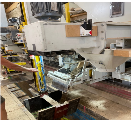
Fig 1: Position of the Dimetix sensor for measuring the height of the tamped clay
